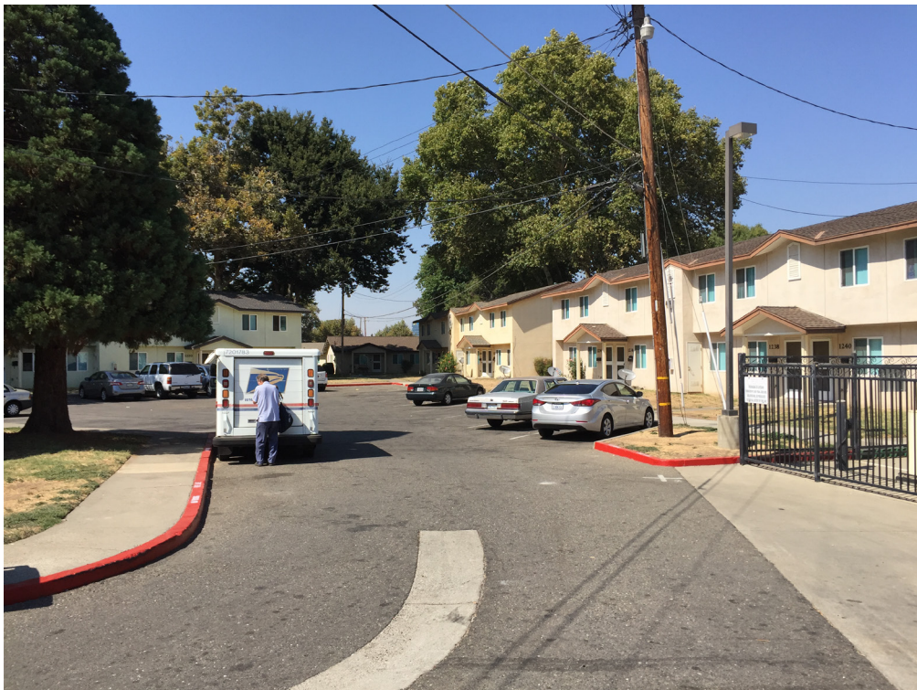
Typical view of internal streetscape within the existing Twin Rivers Community Housing Complex, showing two-story housing units.
